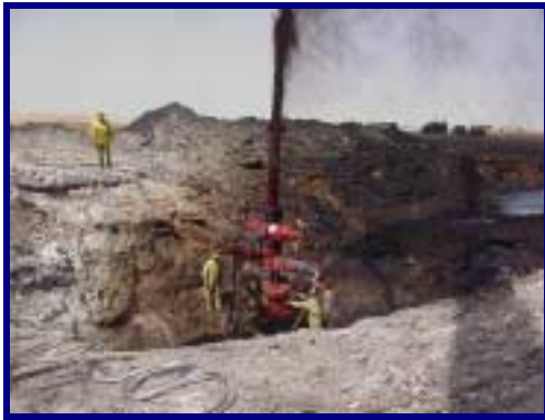
Picture3: capping stack in place
