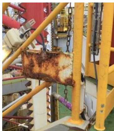
Location of Exit sign
