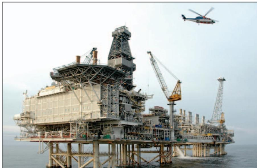
**To combat shallow water flows post cementing on the Azeri-Chirag-Gunashli field, located 100 km east of Baku, Azerbaijan, the drilling team for the Central Azeri Platform applied foam cement on surface casing operations.**
