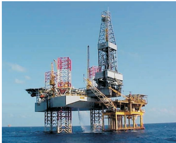
Chiles Offshore ultra-premium jackup Coronado is one of 3 in the company's fleet; 2 more are scheduled to be delivered in 2002.
