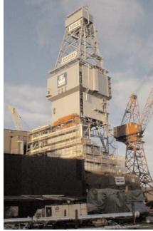
Oseberg Sør: This highly automated rig for offshore Norway is the result of 2 years of design, engineering and fabrication. The unit can operate with a crew 20% smaller than a comparable "standard" rig, manufacturer Bentec says.
