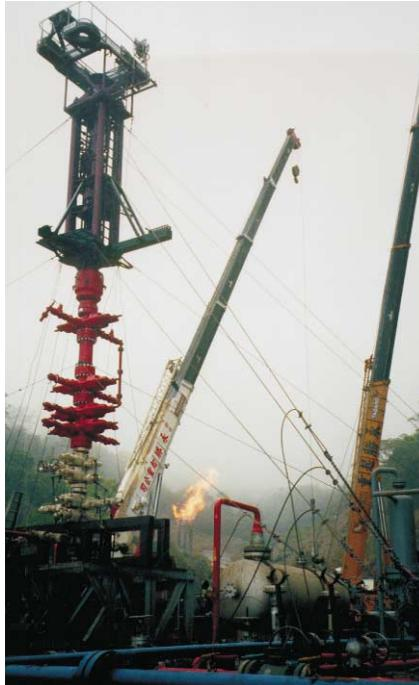
IADC/SPE 59120: The CHK-140W blew out in 1996 at the surface, with the primary broach some 25 m from the well head. The ultimate recovery plan involved challenging snubbing objectives and innovative fluid dynamics.
