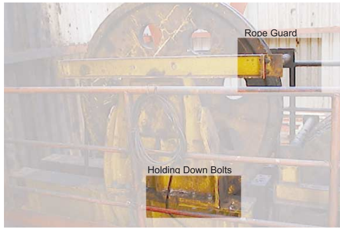
Figure 2: A comprehensive equipment checklist was developed for each area. Photos were annotated as inspection aids to help locate equipment items.
