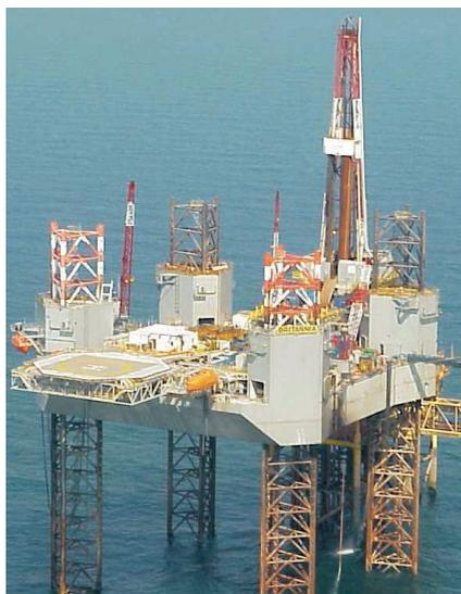
**A large usable deck space area was a key advantage when outfitting the Britannia for underbalanced drilling in the North sea.**
