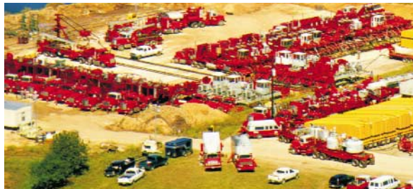
Under threat: A 10-year-old lawsuit alleging drinking water contamination from hydraulic fracturing has brought coalbed-methane operations in Alabama to a virtual standstill. This despite evidence to the contrary, including a comprehensive, independent study of more than 10,000 wells in 13 states. Photo of a hydraulic frac job courtesy of Halliburton Energy Services.
